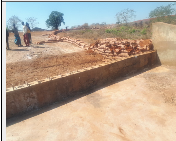
Drop structure at spillway outfall
