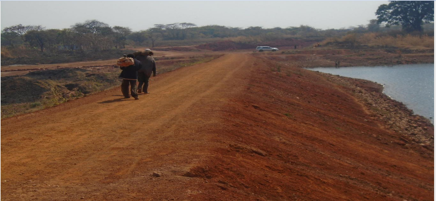
Upstream slope condition – showing variable slopes
