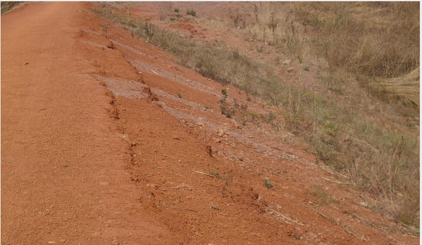
Breakup of downstream crest shoulder and narrowing of Crest
