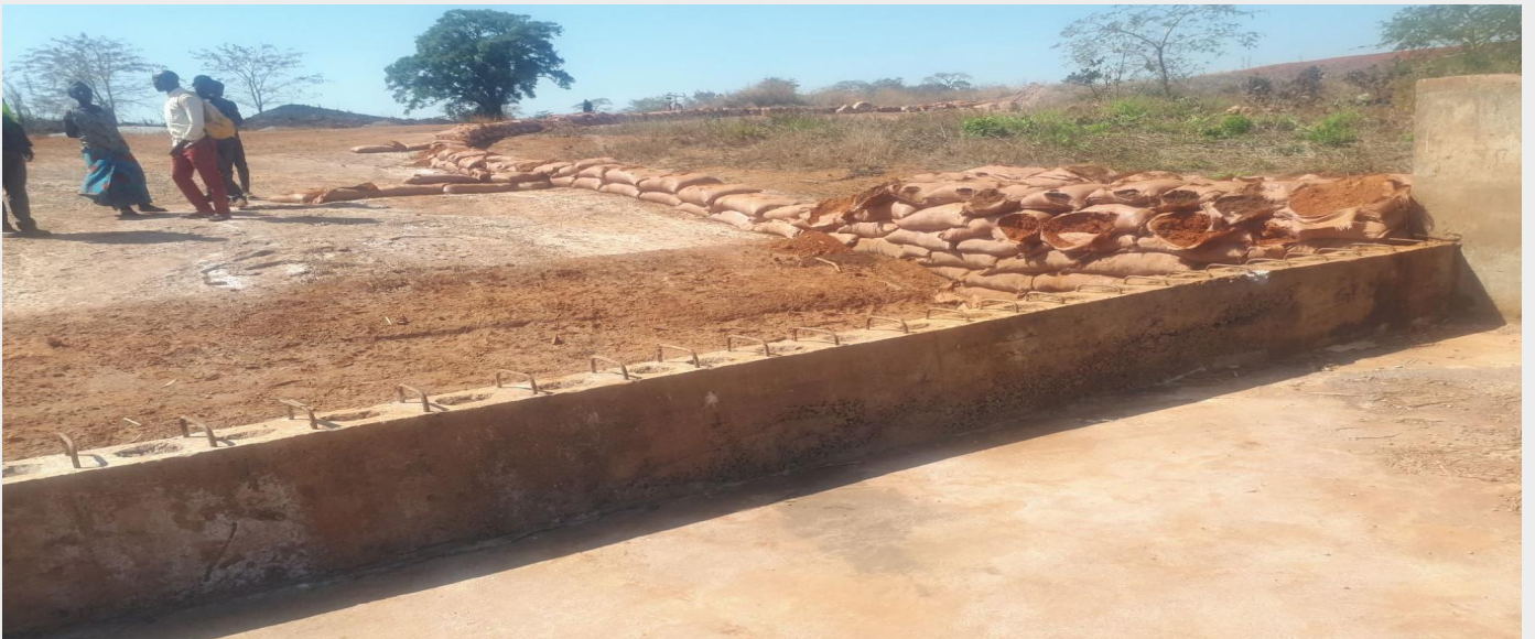
Sandbag training wall from drop structure
