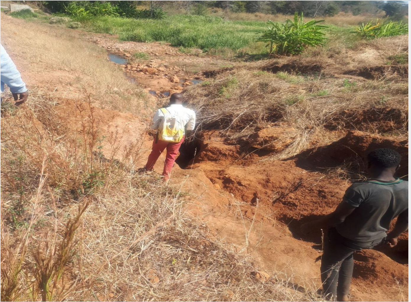
Gully to incorporate in location of new toe drain
