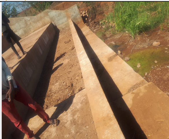
Drop structure near the spillway outfall
