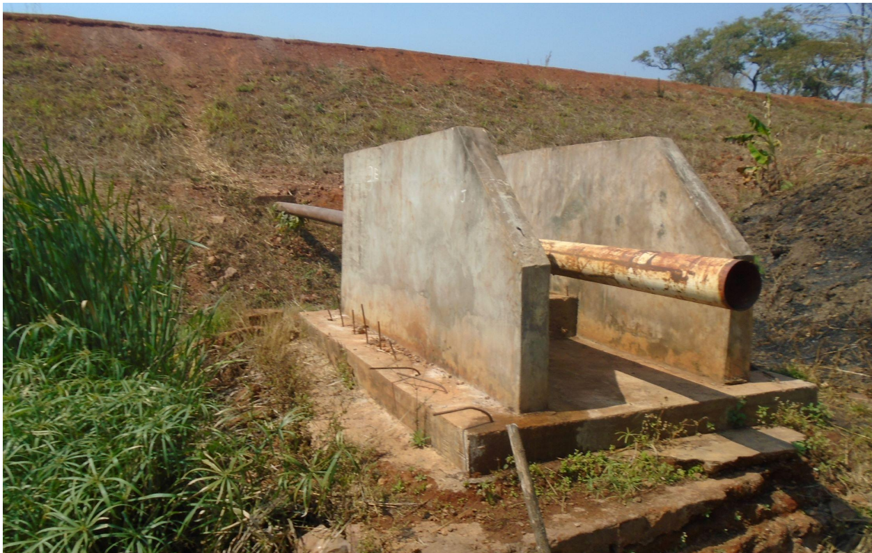
Figure 34 Outlet pipe and valve chamber with seepage point on left
