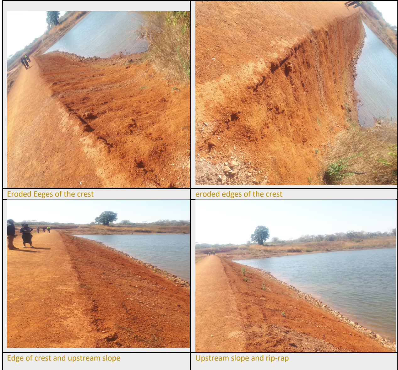
Figure 21 Pictures showing status of crest
