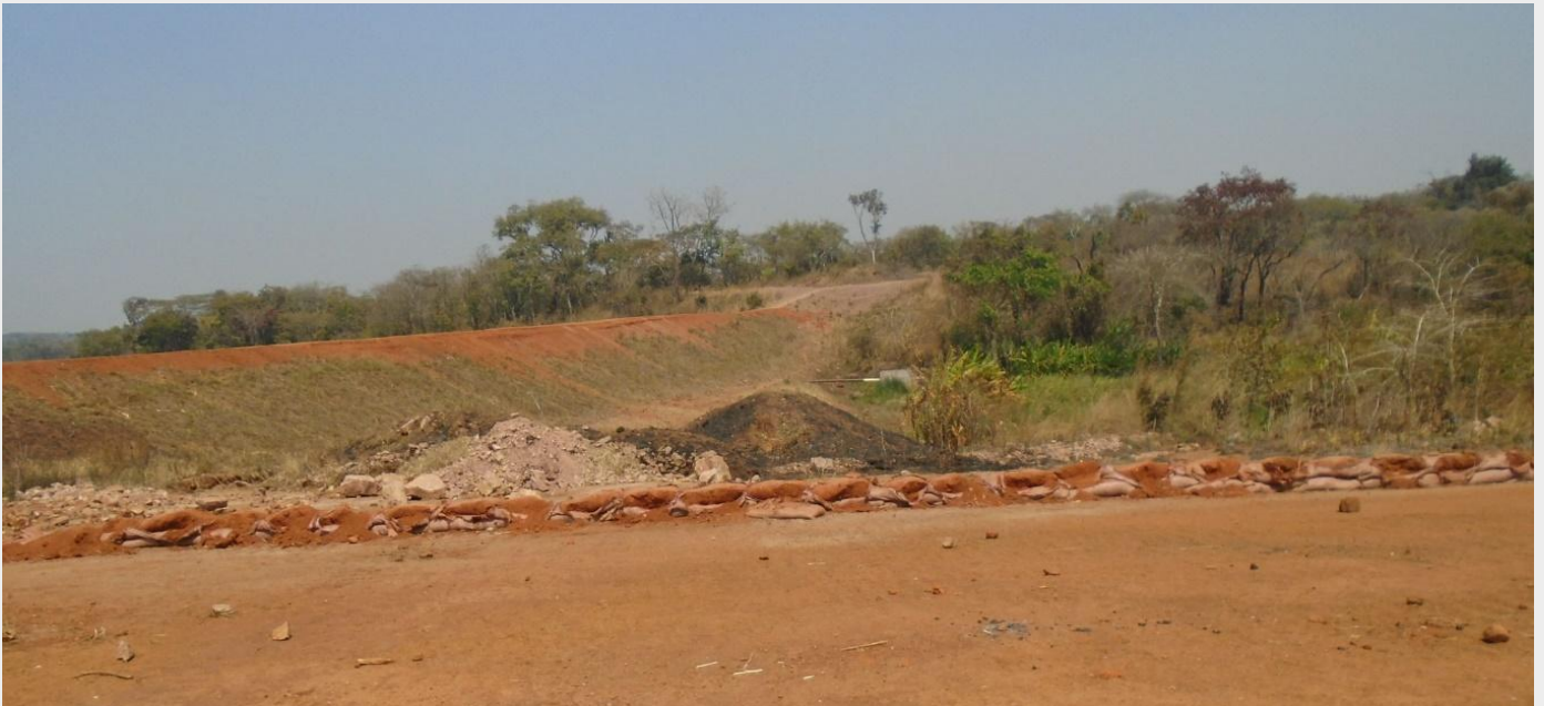
Sandbags forming left bank training wall
