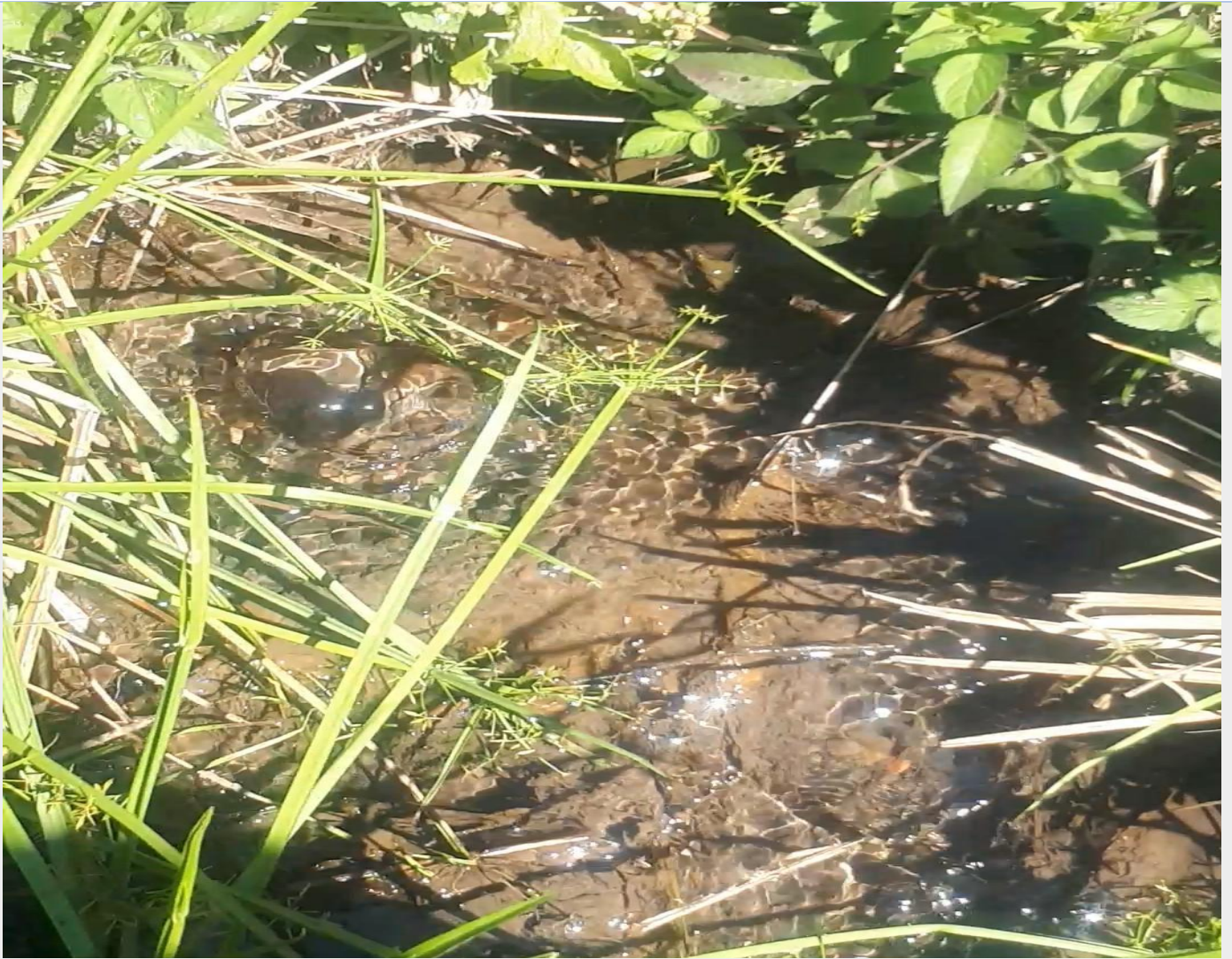
Extensive water “boil” exiting downstream near the outlet
