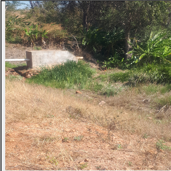
greening due to seepage near the outlet pipe
