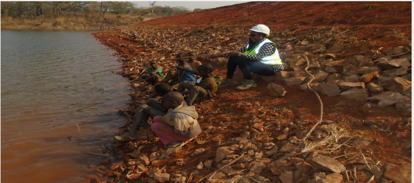
Breakup of rip rap and “Beaching” from wave action
